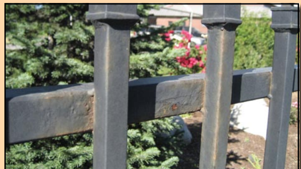
Using unacceptable powder coating - results in fading, discolorization and chipping.
